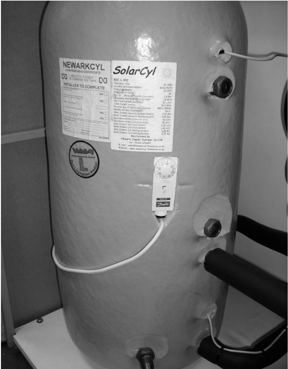
fig 139: cylinder thermostat
