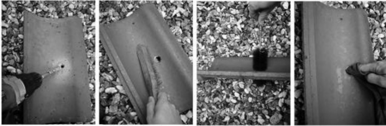
drill tile using pilot bit first up to 18mm hole
