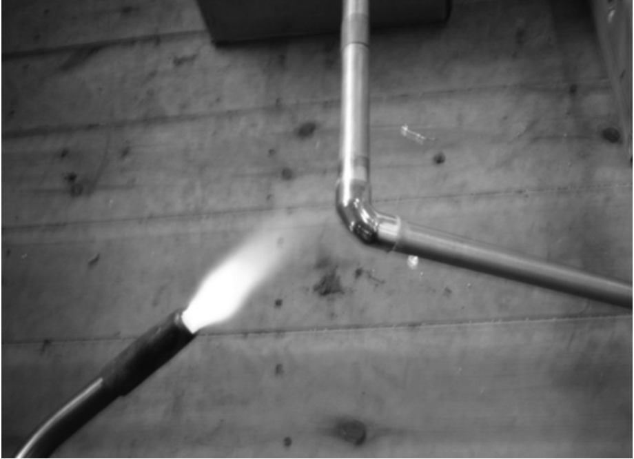
fig 158: soldering pipes
