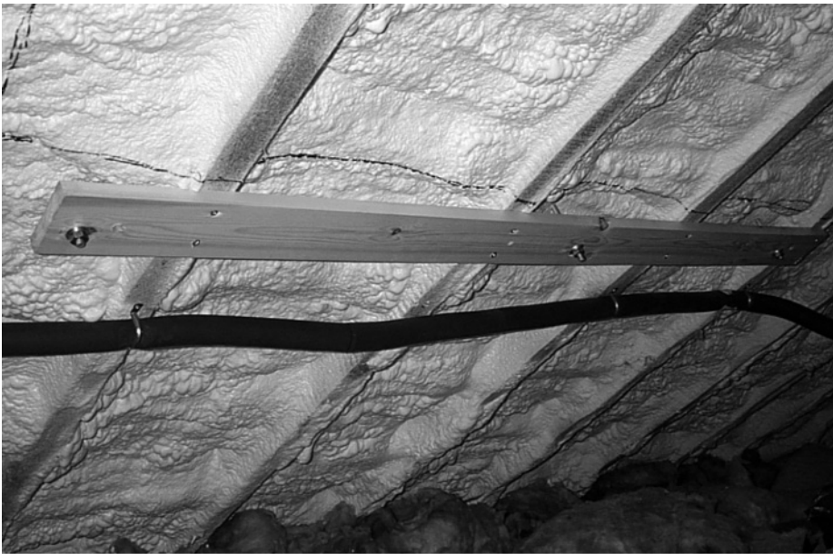
fig 115: fixing batten in the loft space
