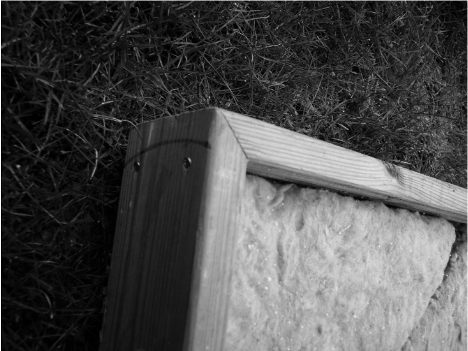
fig 156: mitred corner joint
