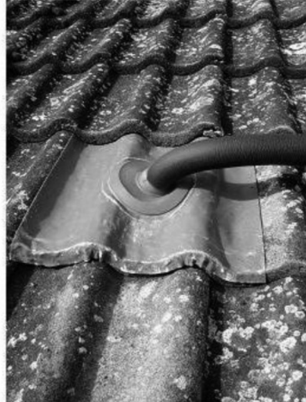
lead soaker with a silicone rubber upstand
