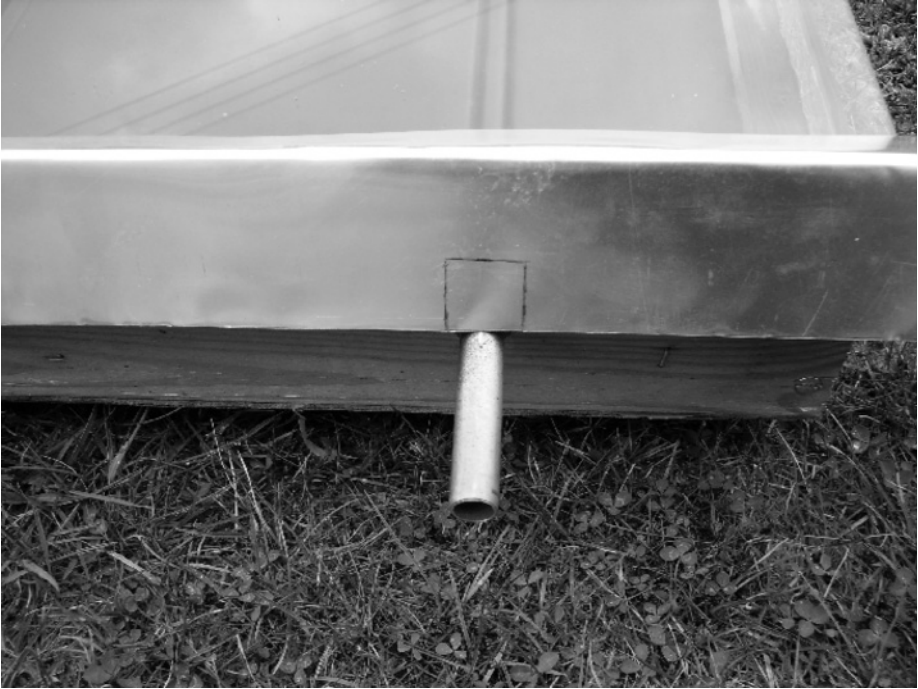
fig 170: ensure the weatherproof trim fits around exiting pipes
