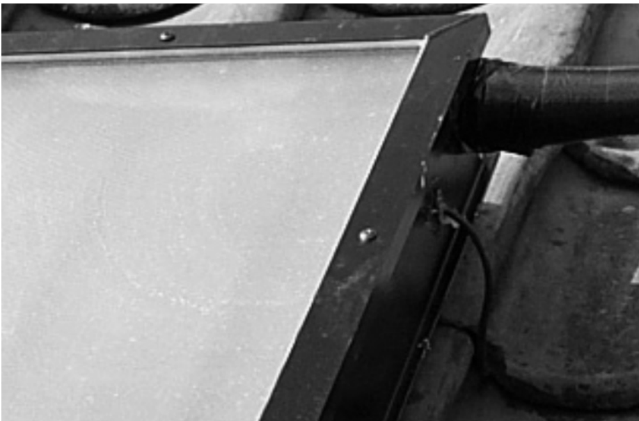
fig 125: Atlas collector sensor connection
