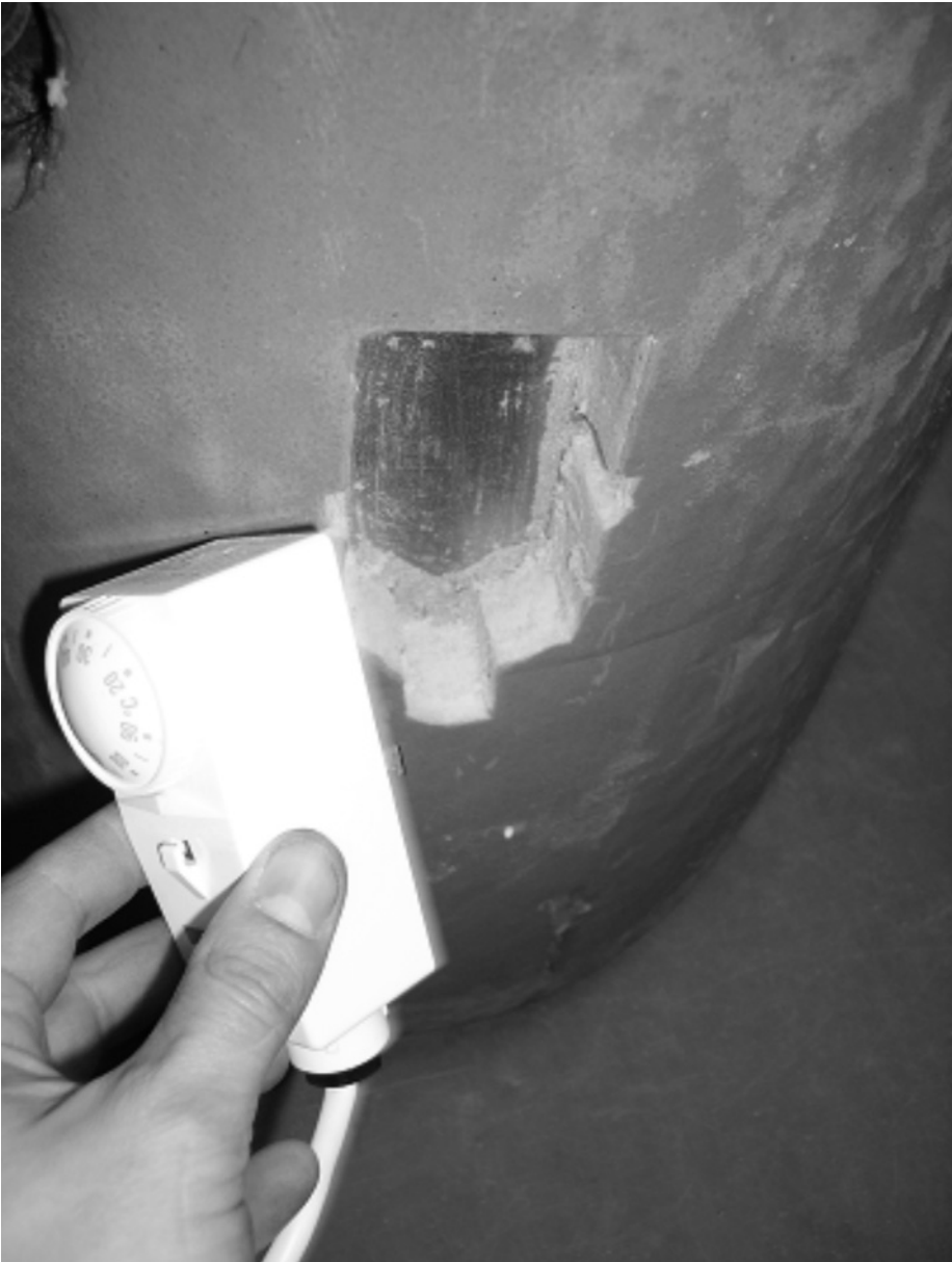
fig 135: removing cylinder thermostat
