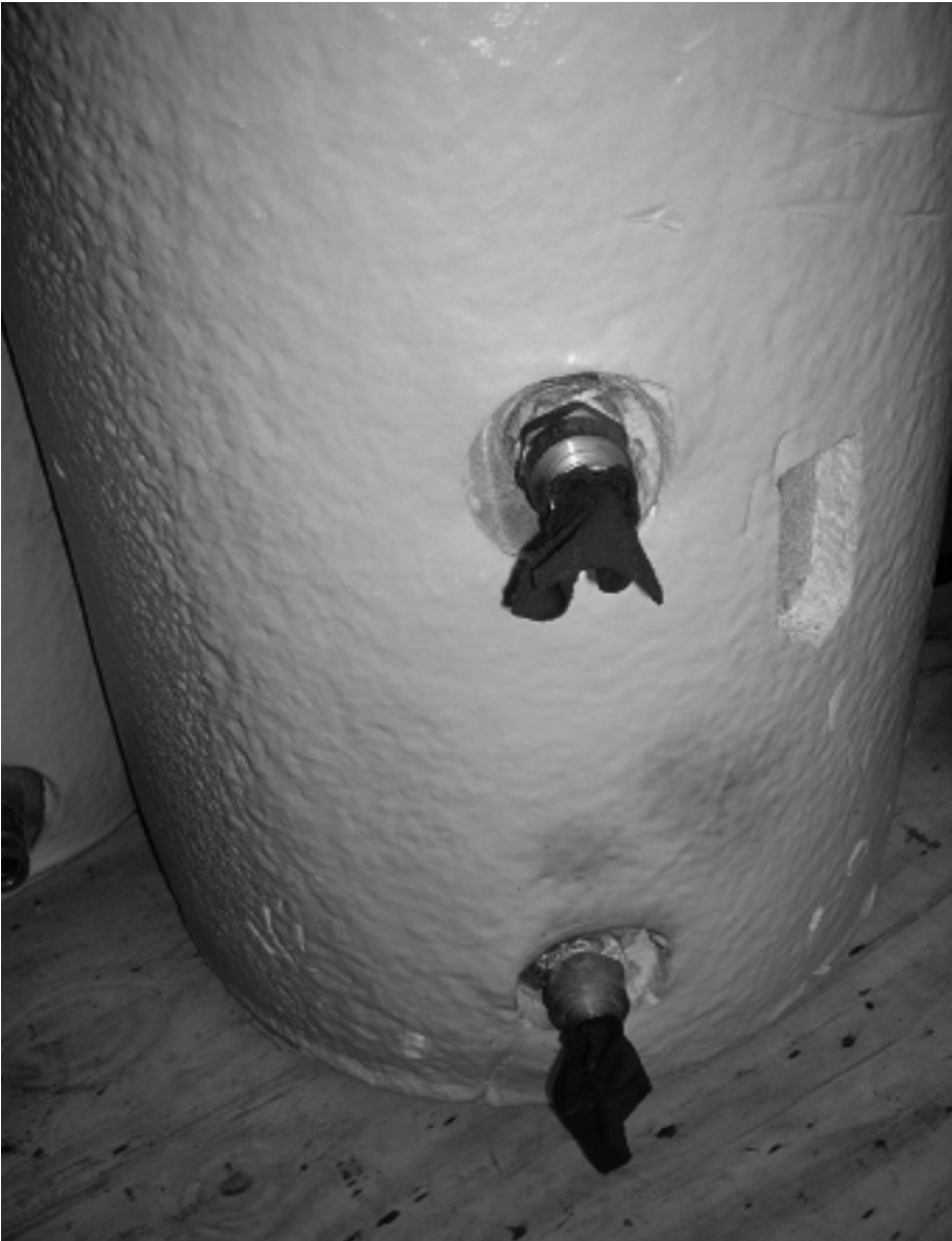
fig 137: the empty cylinder, ready to be moved
