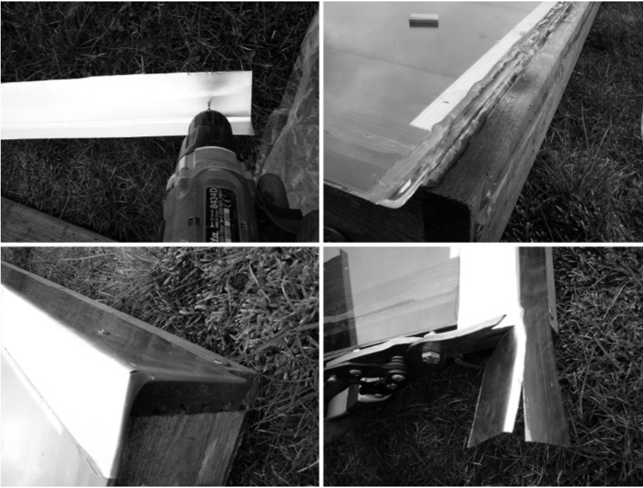
fig 169: fixing the weatherproof trim
