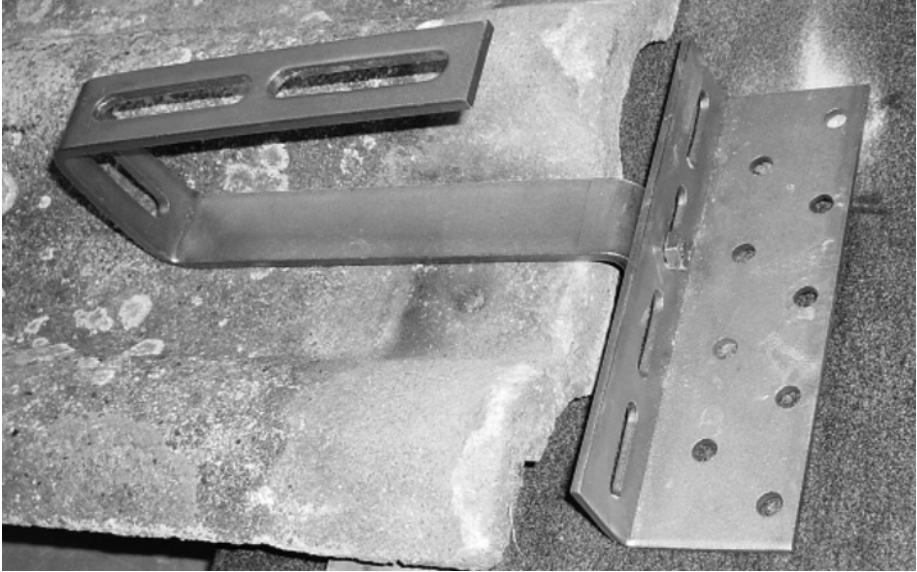
fig 26: hook type bracket with footplate
