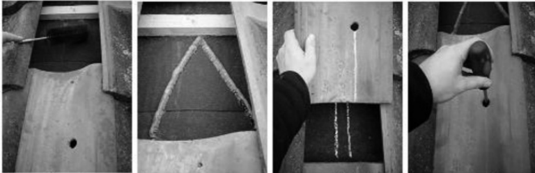
clean felt above drilled tile
