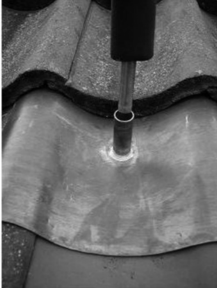
lead soaker with a copper upstand
