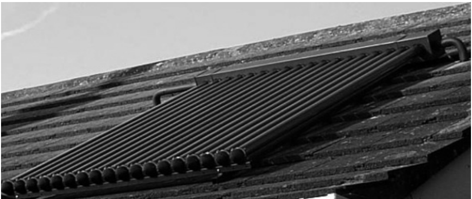
fig 7: glass tube solar panel
