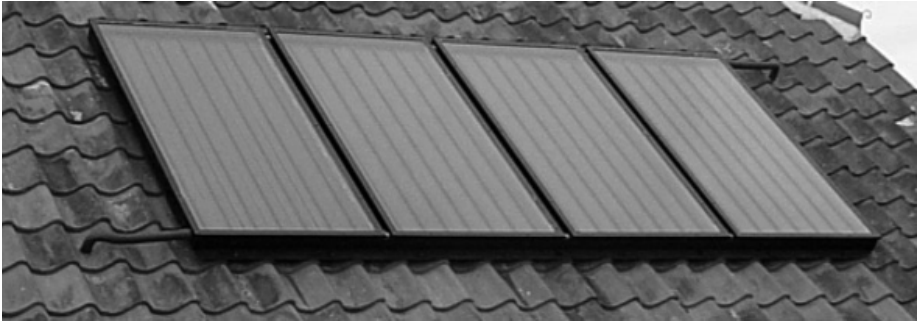
fig 6: flat glass solar panel
