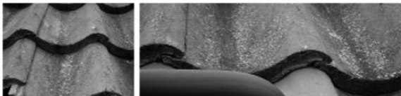
refit surrounding roof tiles
