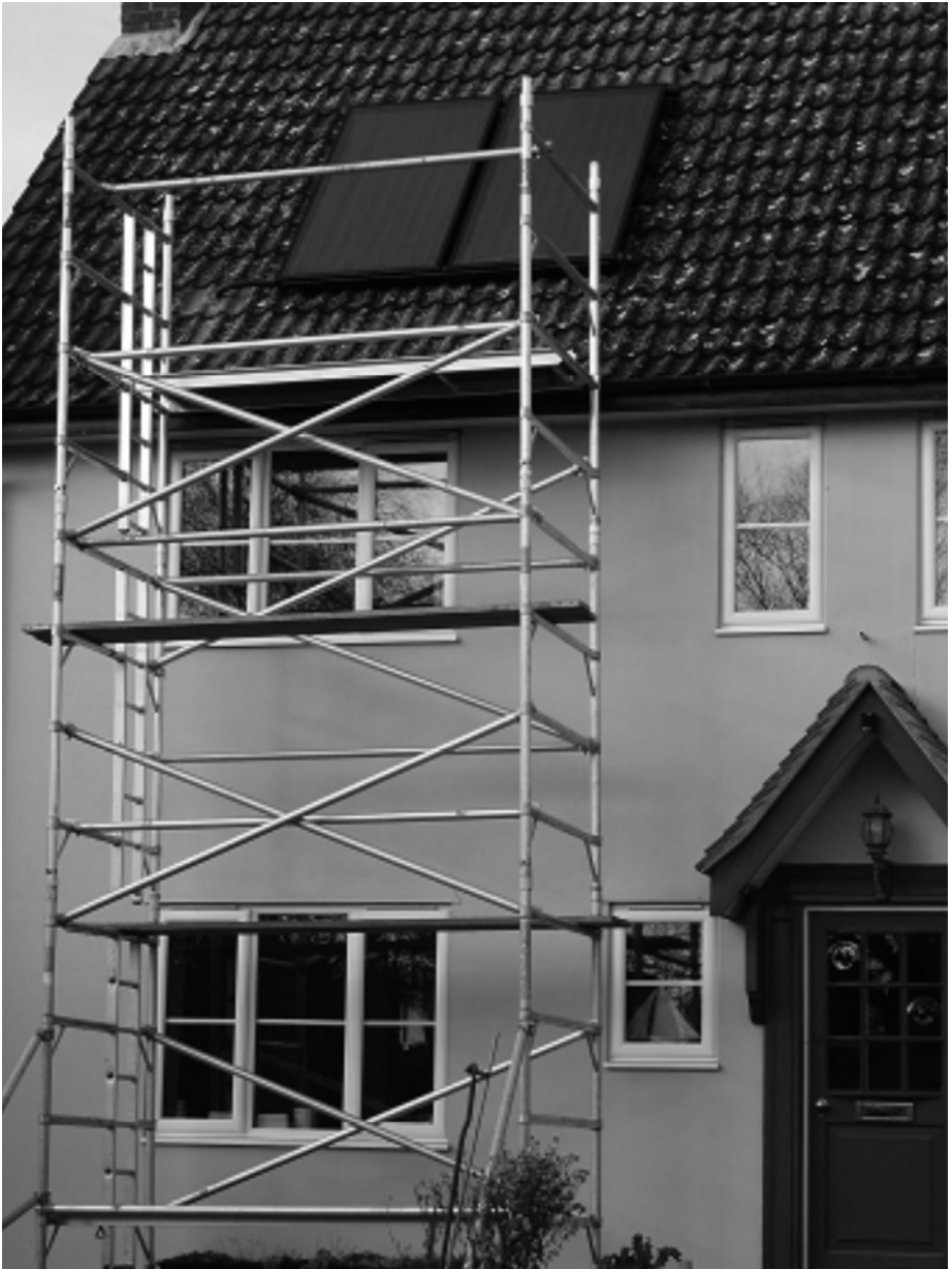
fig 105: mobile platform scaffolding tower
