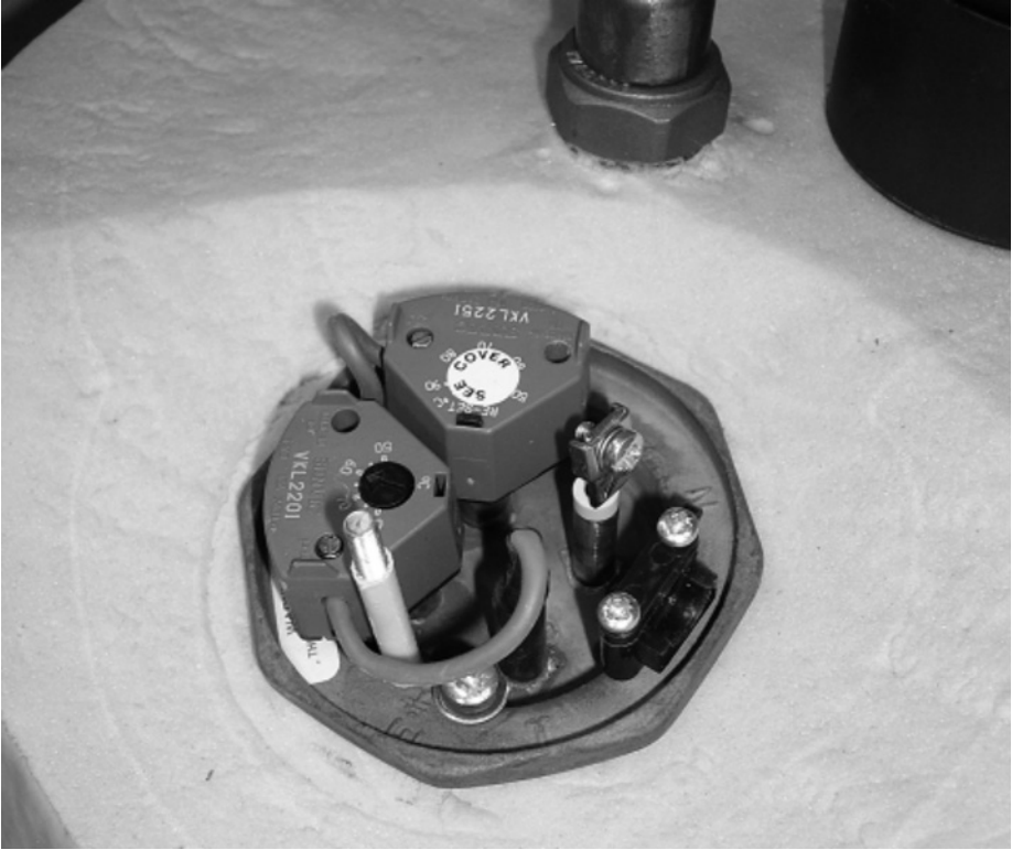
fig 136: disconnect the immersion heater
