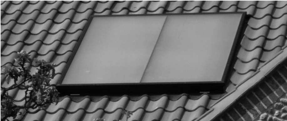
fig 14: commercially produced flat plate collector
