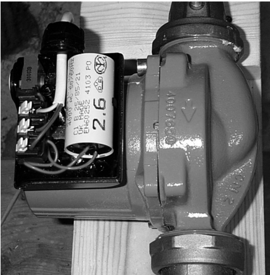
fig 149: pump wiring
