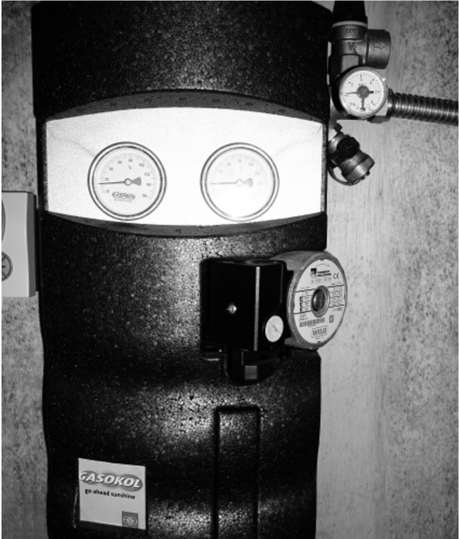
fig 53: completed pump station
