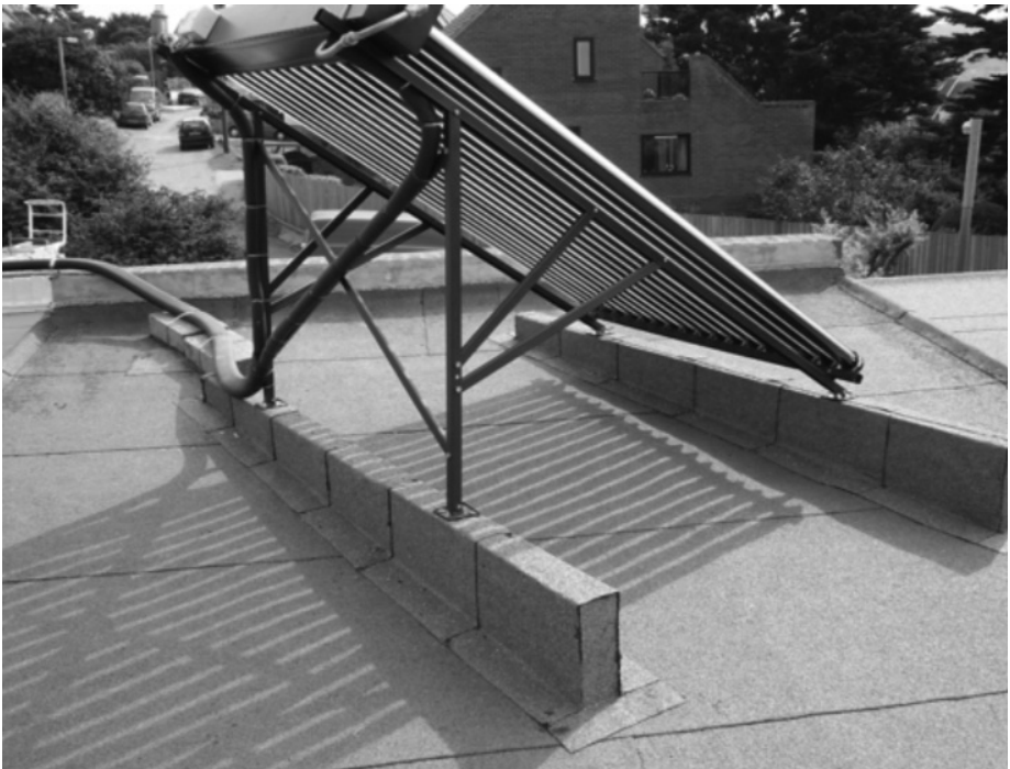
fig 28: collector with horizontal mounting
