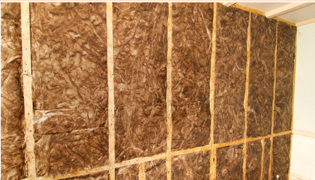
The ThermoShell® IWI system, showing the Earthwool EcoBatts and EcoStuds
