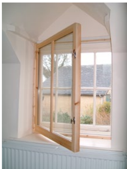
Figure 7.5 Using 4/6/4 mm low emissivity krypton filled glazing gives a high performance for this handmade secondary window. The overall U value is about 1.2 W/m²K. Picture: John Willoughby
