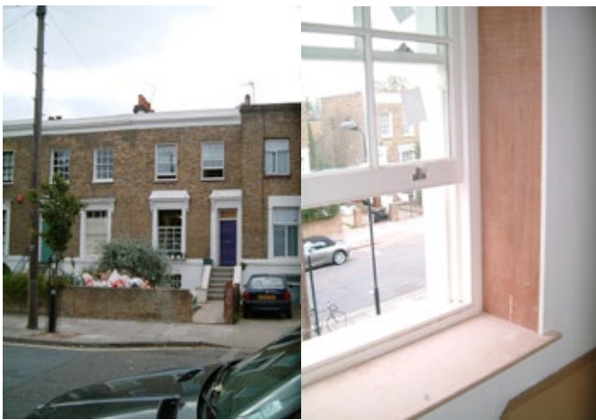
Figure 8.4 Exceptional levels of air tightness have been achieved at this refurbishment project in Hackney. New draught-proof windows have been carefully sealed to new internal wall insulation. Pictures: John Willoughby
