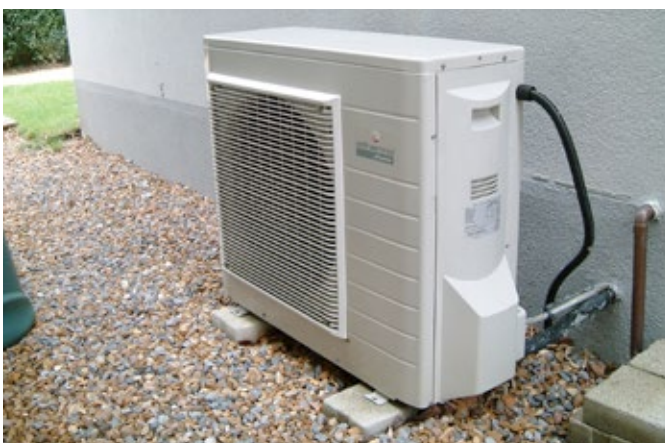
Figure 10.4 An evaporator unit for an air source heat pump. Picture: John Willoughby
