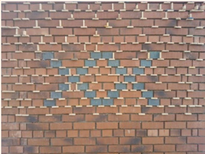
Brick slip installation with spacers
