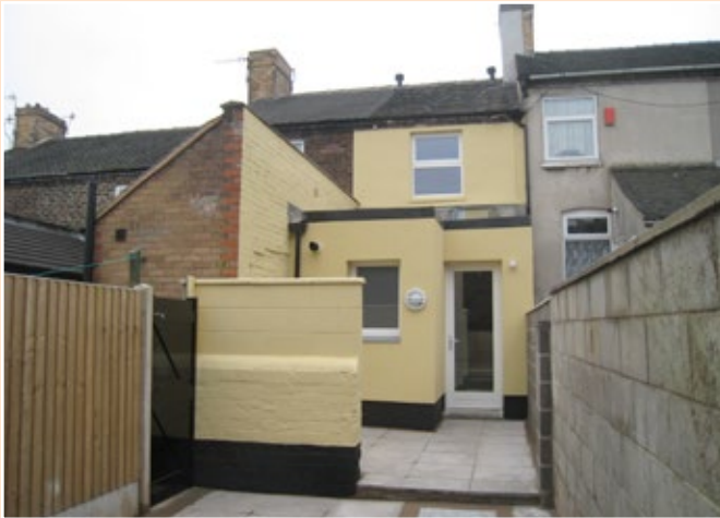
Rear of property after completion
