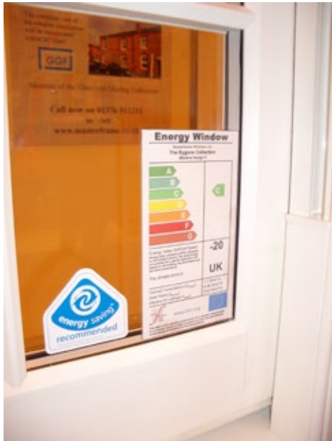
Figure 7.2 Windows are rated on an A to G scale. Picture: Gavin Hodgson, Oxford Brookes University
