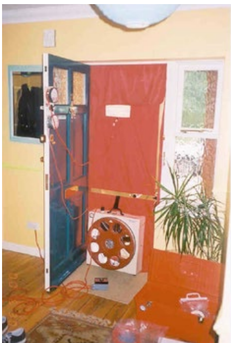
Figure 8.2 Pressure testing equipment. Picture: Rickaby Thompson Associates
