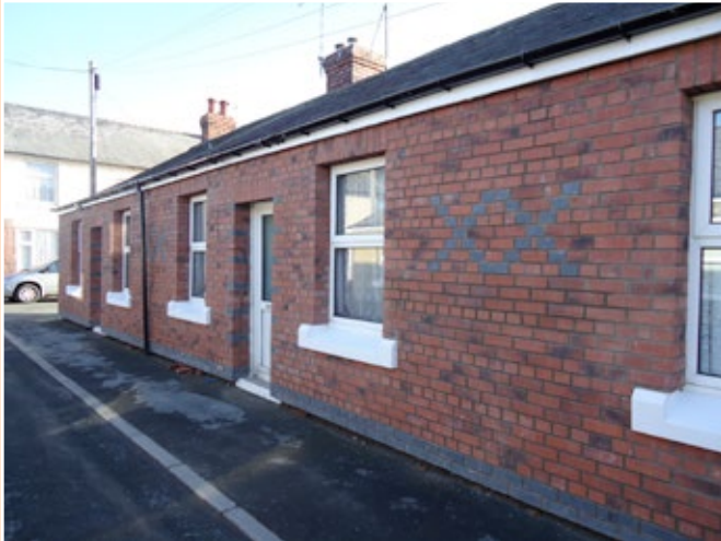
Dee Cottages post works
