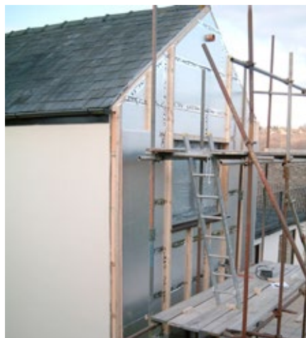
Figure 5.4 Two layers of insulation allow timber battens to support the extended roof verge. Picture: John Willoughby
