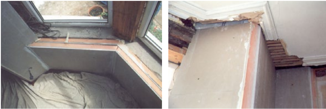
Figure 5.15 Internal insulation at the Nottingham EcoHome. Pictures: Gil Schalom
