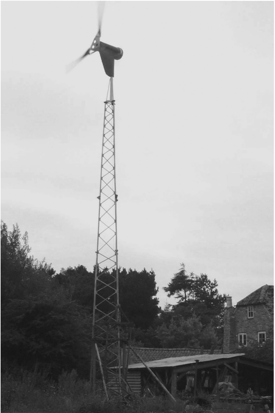
fig 67: Proven 2.5 kilowatt turbine on a 15 metre mast
