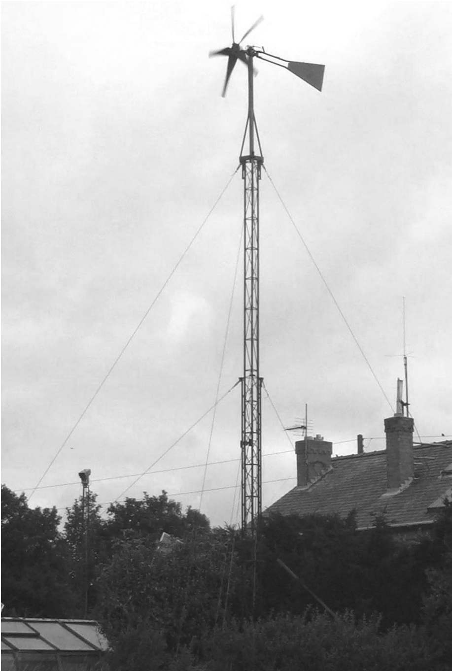
fig 66: FuturEnergy 1 kilowatt turbine on a 12 metre mast
