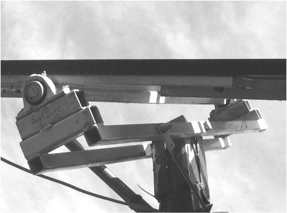
fig 30: panel sub-frame and bearings
