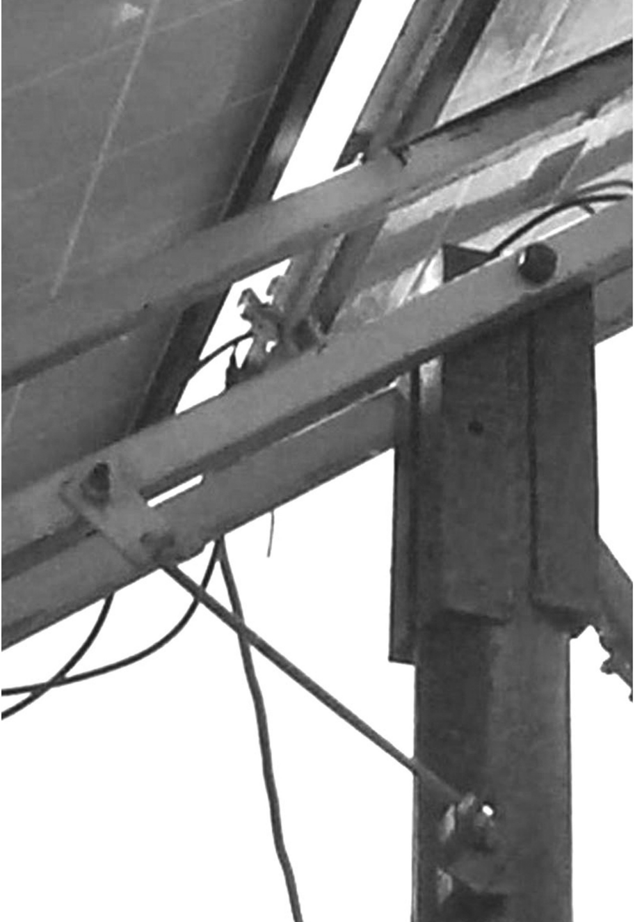
fig 27: angle adjustment mechanism for pole-mounted system
