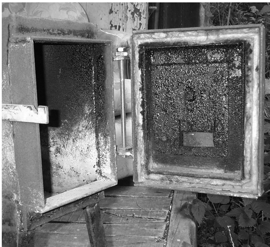
fig 49: doorframe, door and seal
