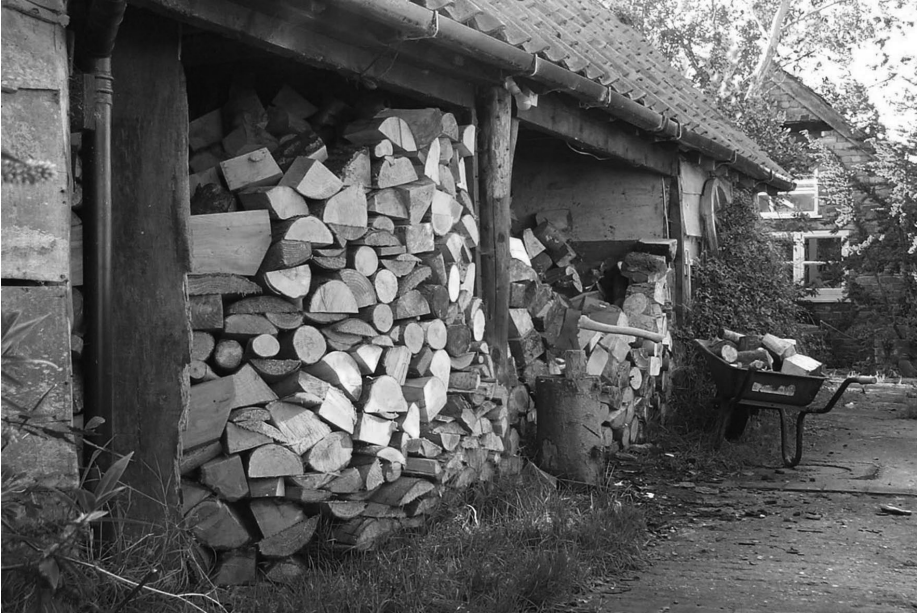
fig 5: wood sheds with plenty of ventilation for drying.
