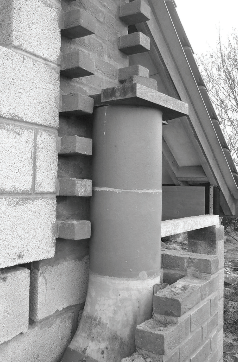
in the new brick chimney may be more appropriate. These are ceramic
