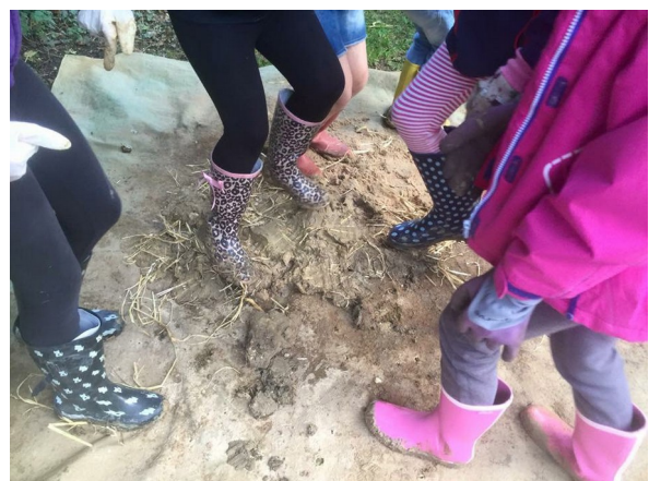
Mixing clay and straw for daub.
