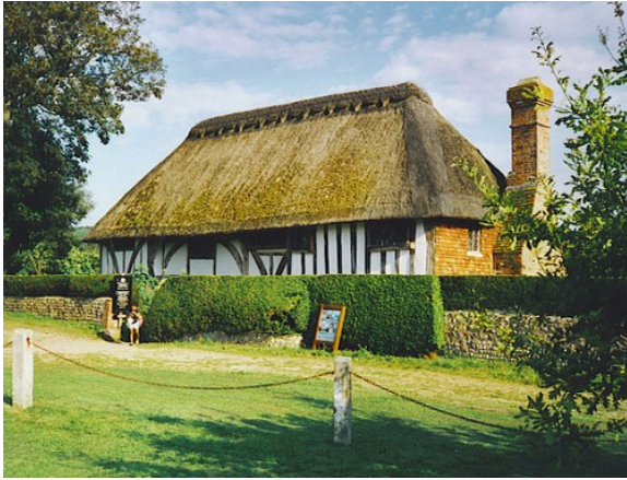
Alfriston Clergy House, in Sussex, UK, has original wattle & daub panels almost 700 years old.
