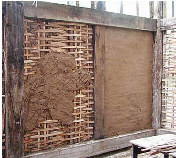
Timber-framed building with panels at various stages of wattle & daub infill.
