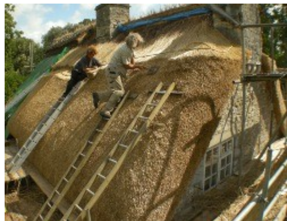
Thatchers at work on a roof.
