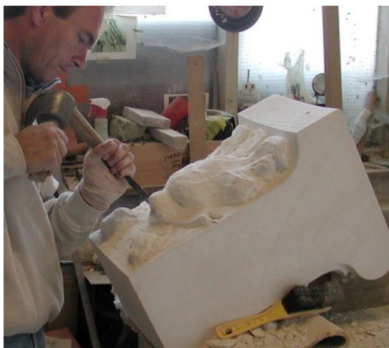
Stone carver repairing stone decorations for Canterbury Cathedral.
