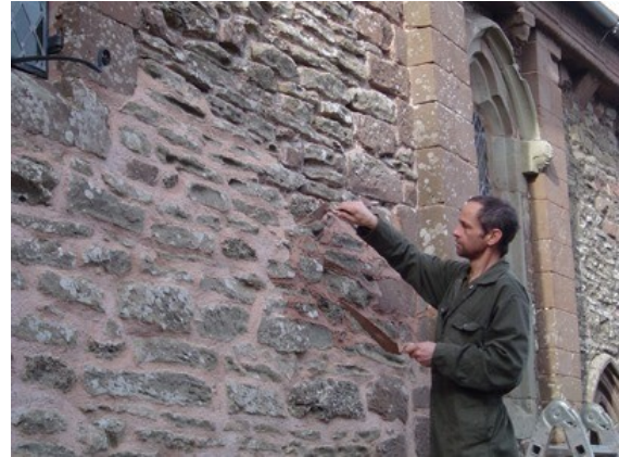
Repointing a stone wall with lime mortar.
