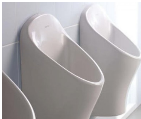
Waterless urinals don't use mains water to flush, and can divert urine to be diluted (or composted with straw, sawdust etc.) and used as fertiliser.
