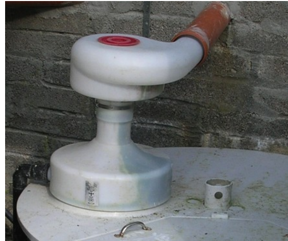
Aquatron separator unit for faecal separation and composting.
