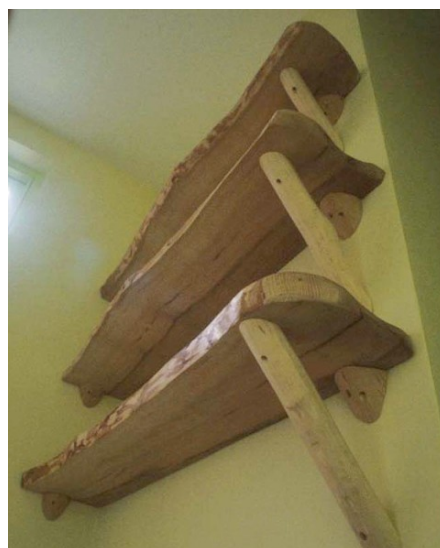
Shelves made from rough-sawn timber and tree branches.
