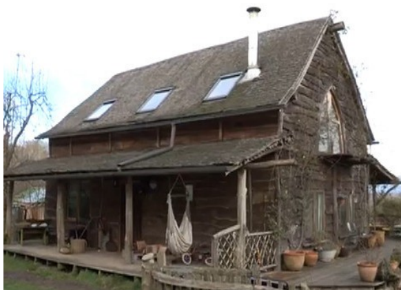
Ben Law's self-built, round wood timber frame house in the woods in Sussex.
