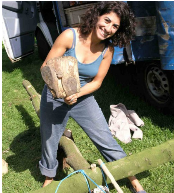
Hammering a peg into a round wood joint with a home-made wooden mallet.
