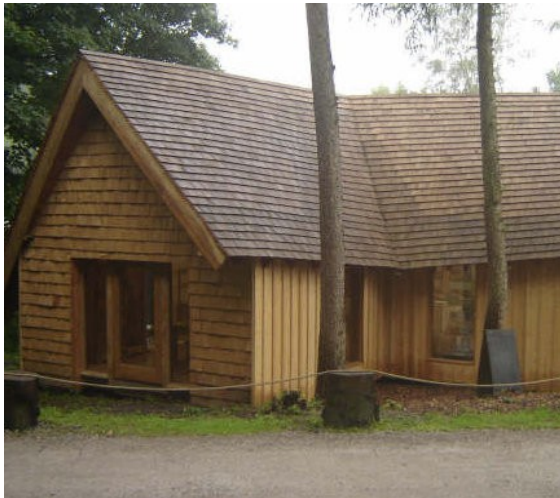
A building in Sheffield with oak shingles on the roof and walls.
