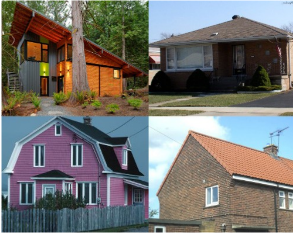
Roof types (clockwise from top left): single-pitch or lean-to; hip; double-pitch; gambrel.
