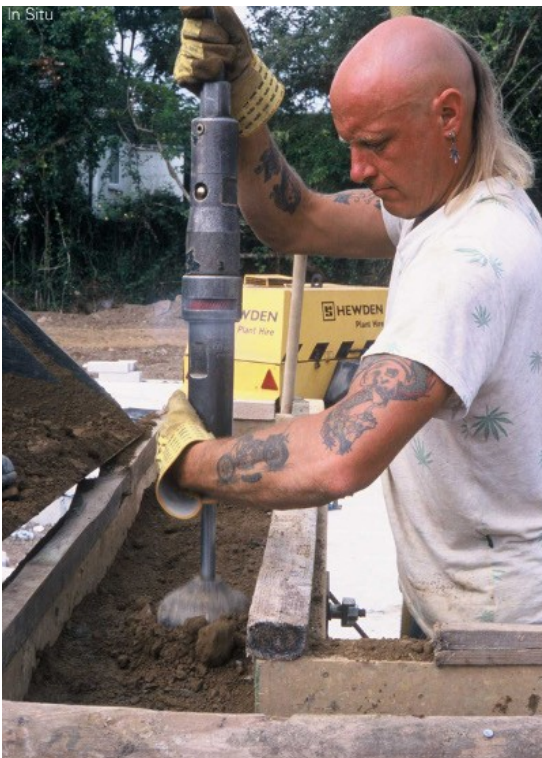
Compacting earth into formwork with a pneumatic ram to construct walls.
