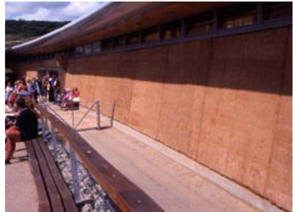
Eden Project: this wall at the Eden Project in Cornwall was built of rammed earth by Rammed Earth Consulting (see resources).
