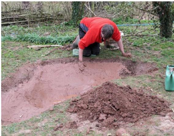
*Pond being constructed with puddled clay.*
