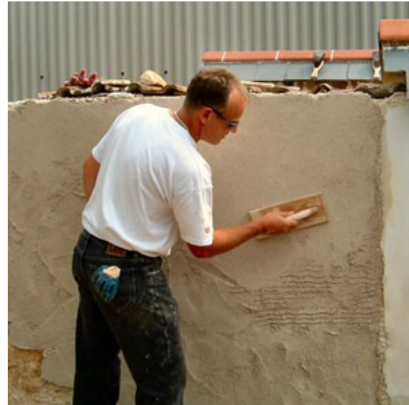
Applying a lime render to an external wall with a float.
