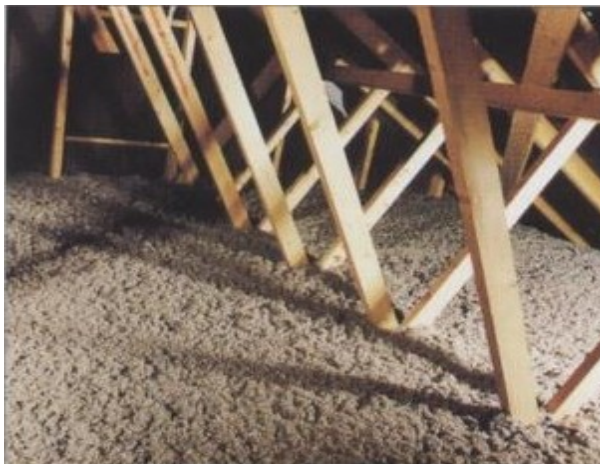
Warmcel - recycled newspaper, loose-fill insulation - poured into a loft.
