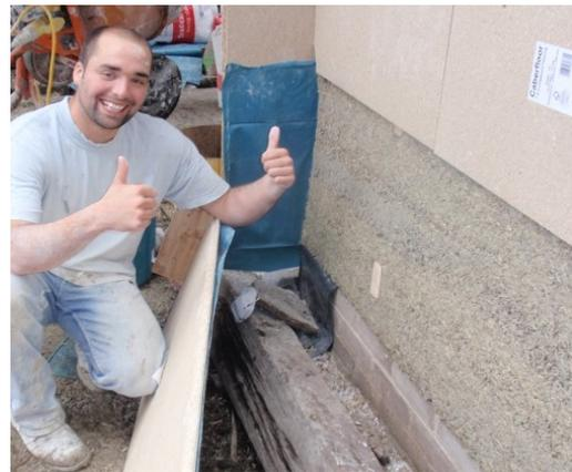
*Removing the shuttering to expose a raw hempcrete wall.*
