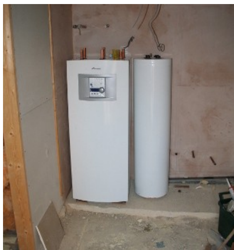
The heat pump itself is the size of a fridge-freezer, with a smaller buffer tank next to it.
