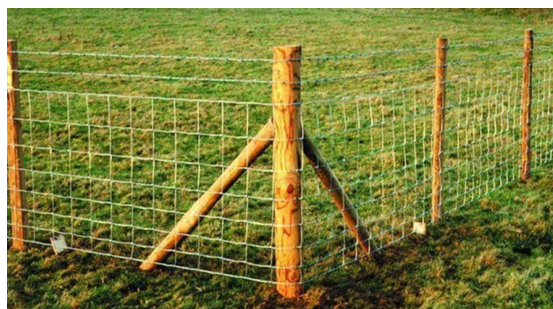
Corner of sheep fence, with straining post and two bracing posts.
