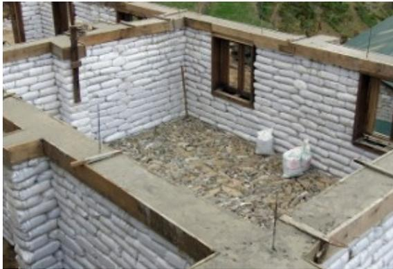
*Earthbag building in Nepal with cement bond-beam in place. (timber would be more usual in eco-builds).*
