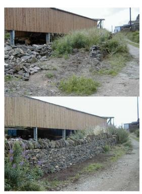
Dry stone wall before and after repair.
