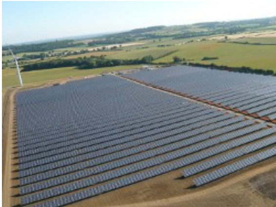
20,000 solar panels covering 30 acres on the Oxfordshire / Wiltshire border, owned by Westmill Solar Co-op
