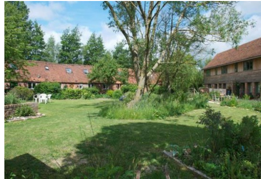
Central area of the Threshold Centre in Dorset, with 14 units, 7 in shared ownership with a local housing association.
