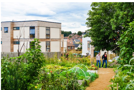
LILAC in Leeds is a 20-household cohousing new-build using the new 'mutual home ownership society' model. The buildings are of straw-bale and timber.
