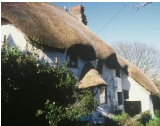
Traditional thatched cob cottages in the south-west of England.
