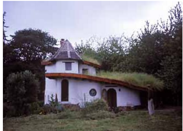
A modern cob home with living roof, in the US.
