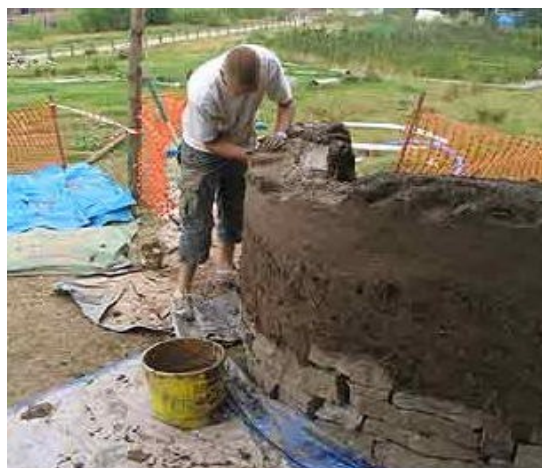
Building a cob wall, mud-pie style.
