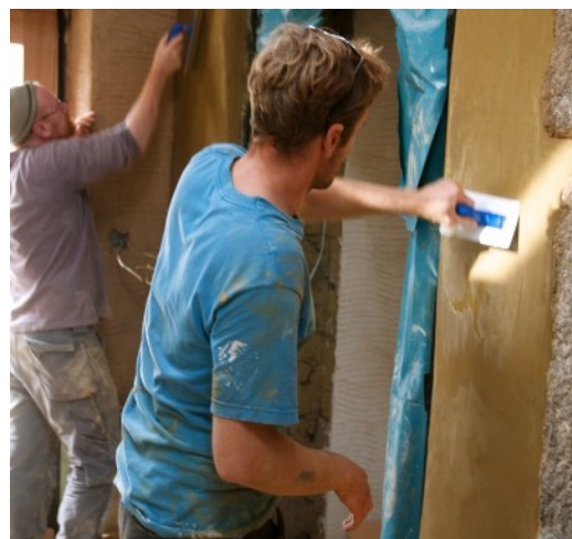
Clay plasterers hard at work.
