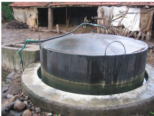
Biogas digester on a family farm in India; there's no reason they can't be successful in the West too.
