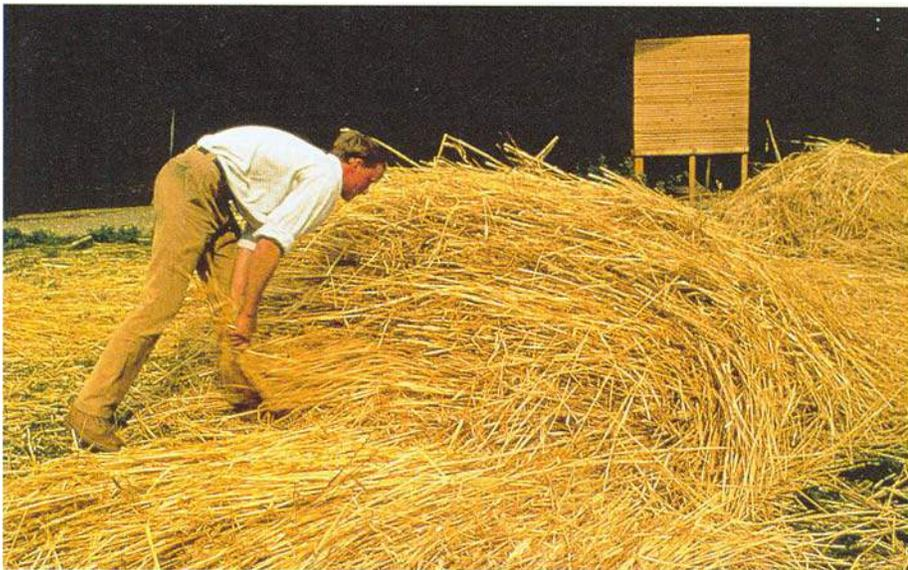
Fig 13 Drawing straw (Photograph copyright @ John B Letts)
