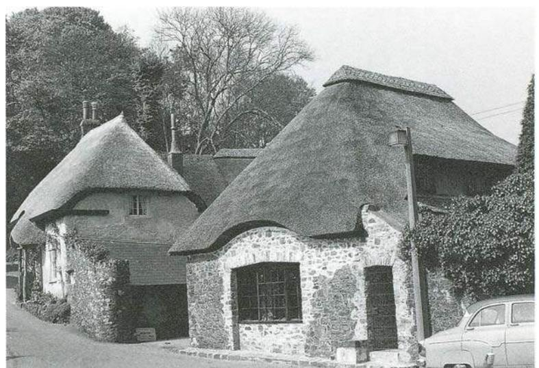
Fig 5 By contrast, the house in Devon (background) roofed in the same material, shows the more rounded outline of a typical hipped Devon roof thatched in combed wheat reed. The house in the foreground is thatched in water reed. (Photograph copyright @ Rural Development Commission)
