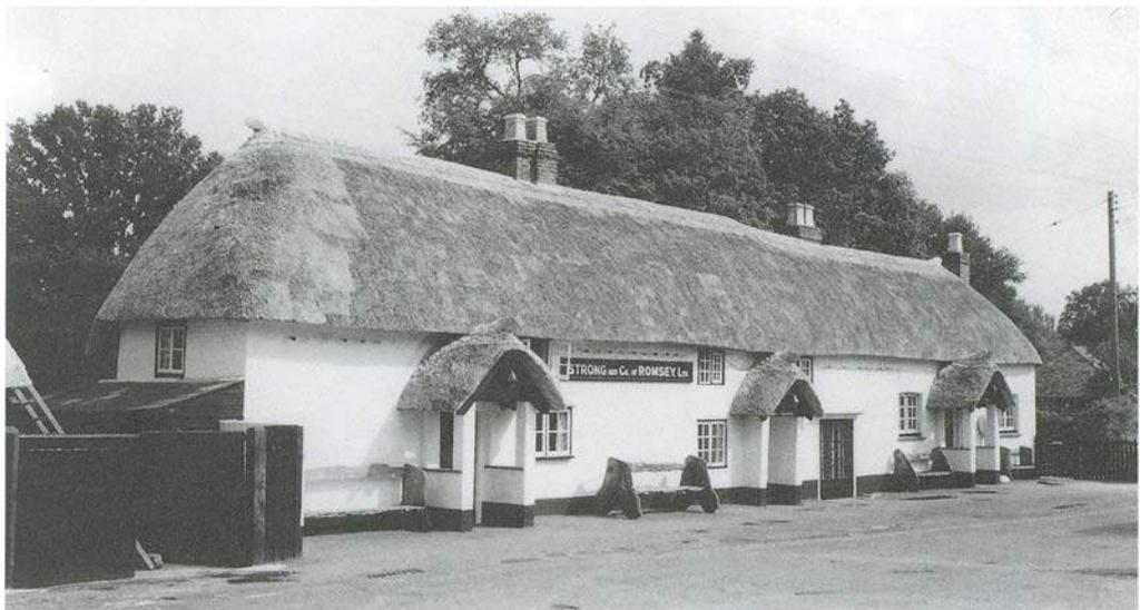
Fig 22 How the character of a building can be affected by re-thatching. The Sir John Barleycorn some years later with a combed wheat reed roof. (Figs 21 and 22 both copyright @ the Rural Development Commission)
