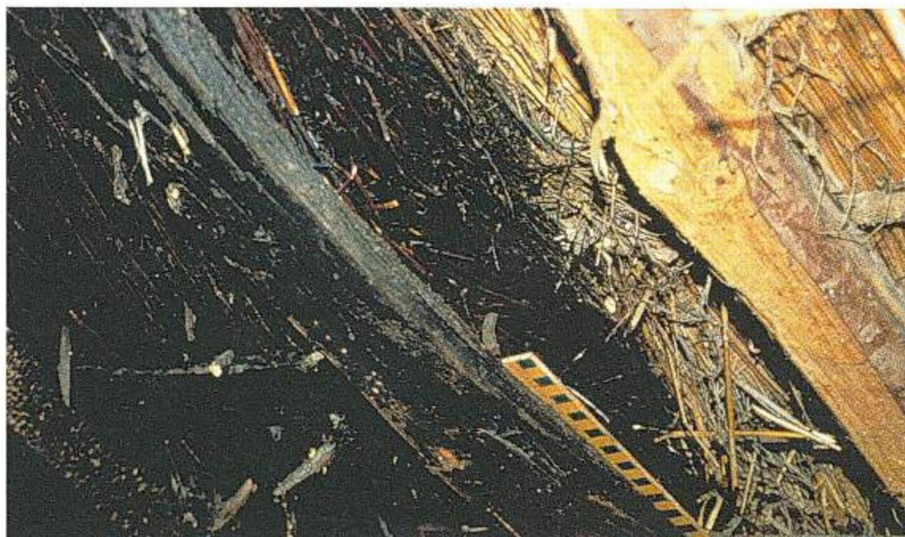
Fig 3 Smoke-blackened roofspace. In this photograph the contrast is clear between the sooting of the earlier portion of the roofspace (left), and the later part (right) which was built after the house ceased to have an open fire. (Photograph copyright © John B Letts)
