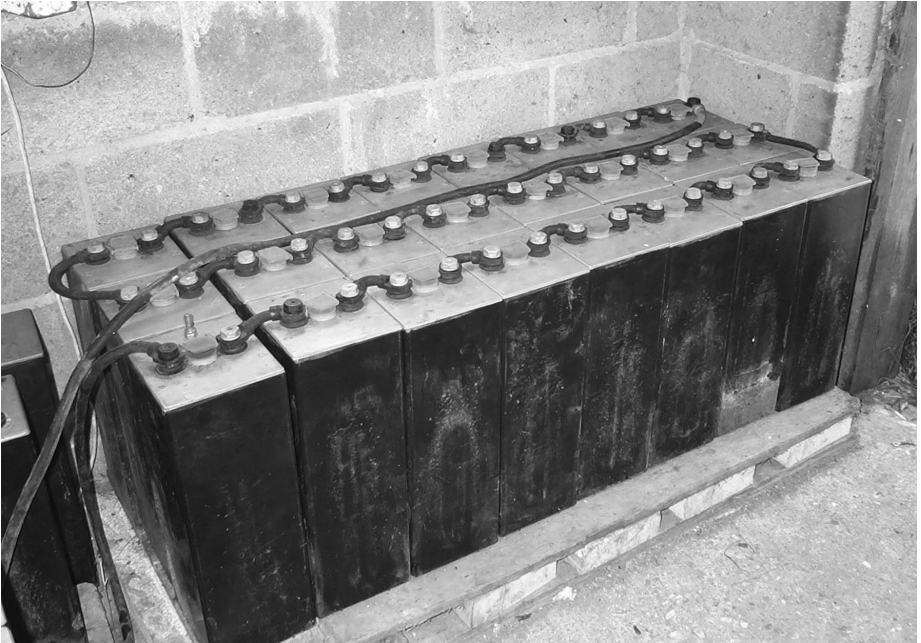
fig 55: battery bank
