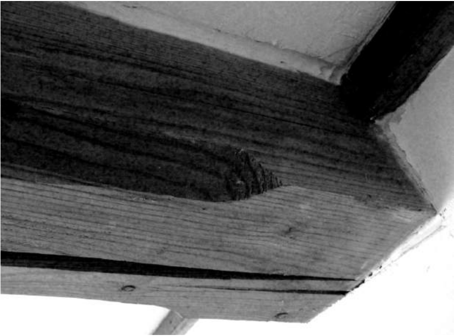
fig 92: stopped chamfer
