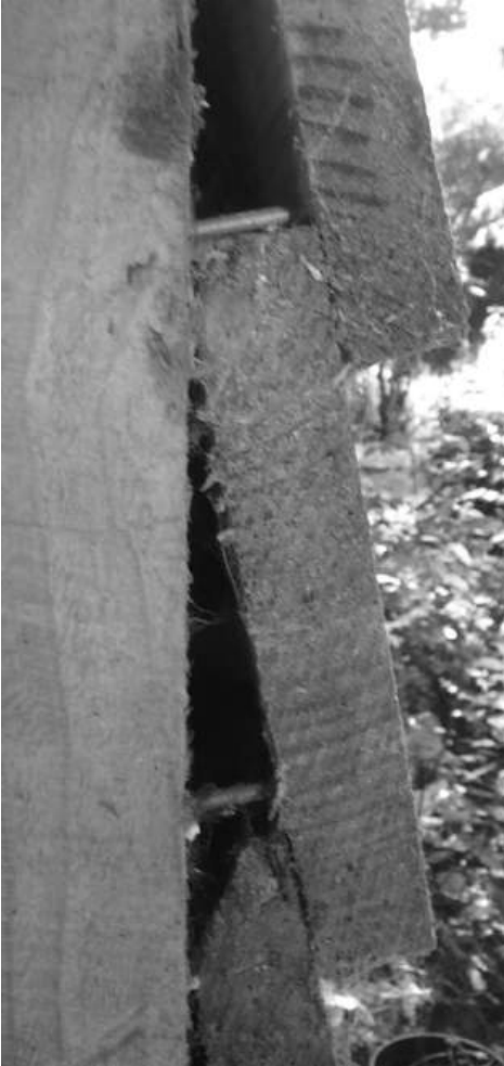
fig 77: weatherboard nailing
