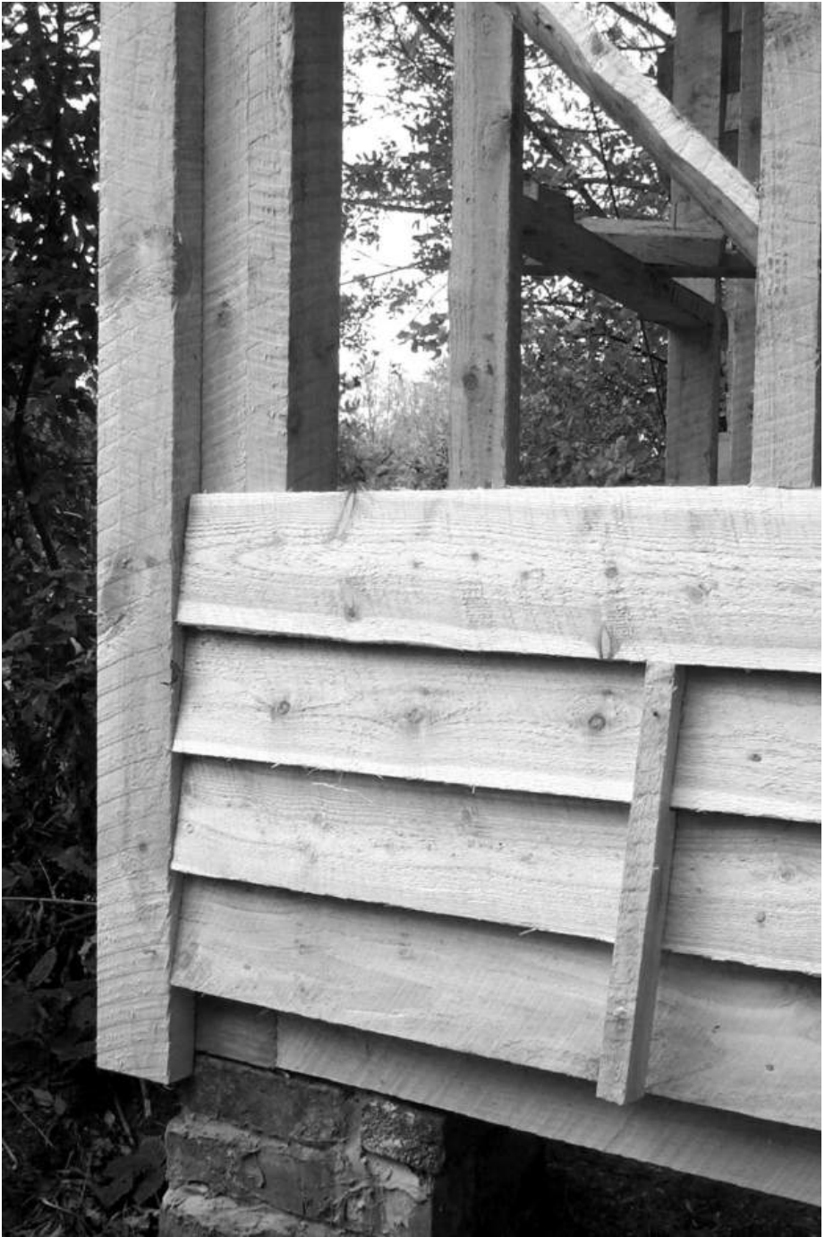
fig 66: home-milled weather boards.
