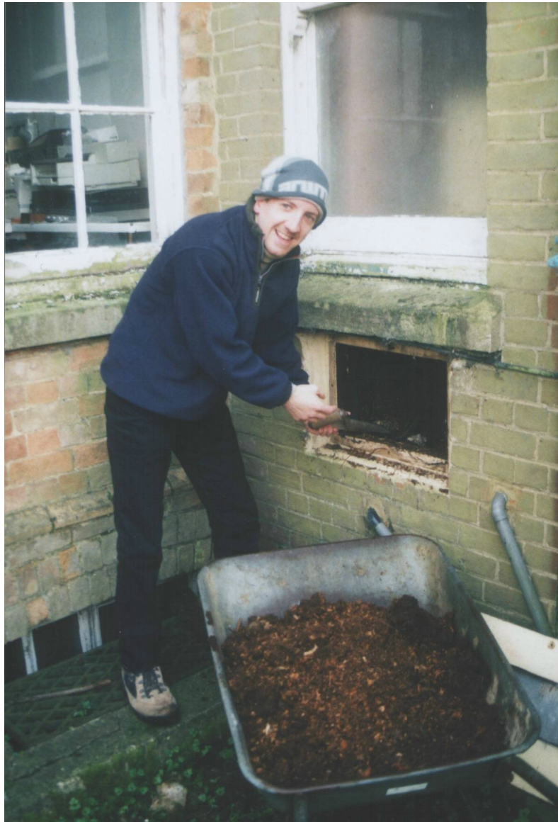
Emptying the 'rested' chamber with a long-handled shovel into a wheelbarrow, for use on our apple trees.
