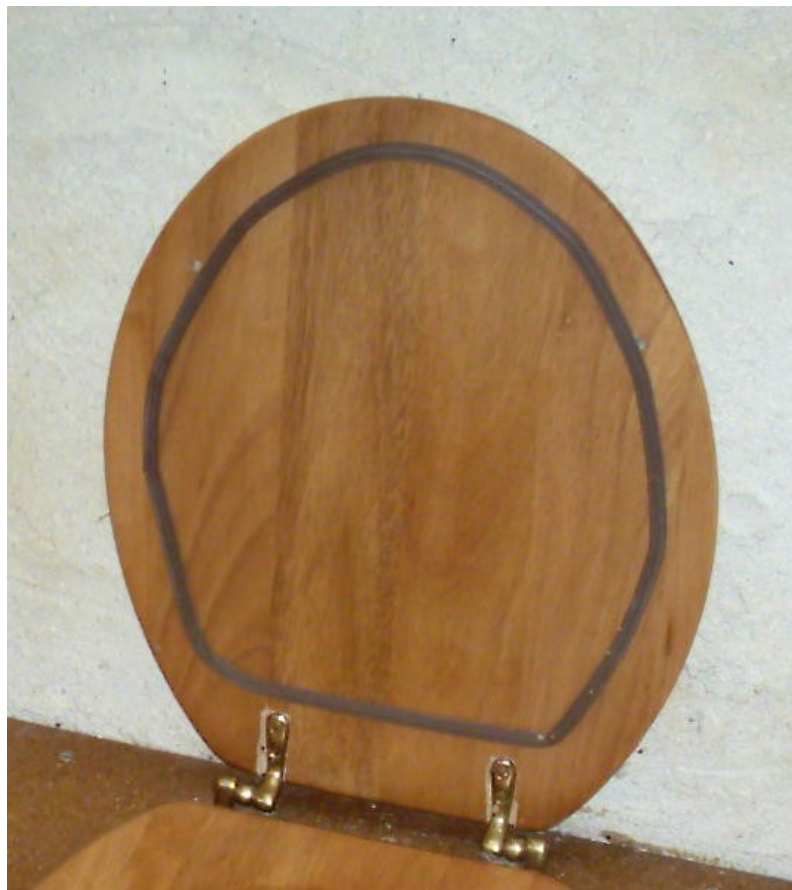
Here you can see a ring of draught-excluding strip around the lid, to stop smells venting into the room, and to stop flies entering.
