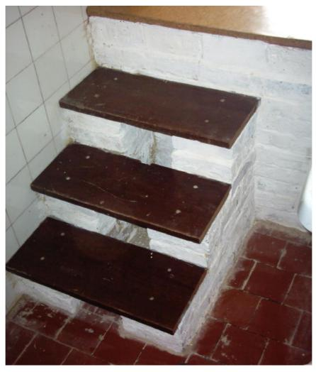
These steps are made from bricks with recycled timber treads. We calculated the optimum dimensions for people to be able to step up to the platform comfortably (see drawing). The bricks were laid with lime mortar and painted with a lime wash.
