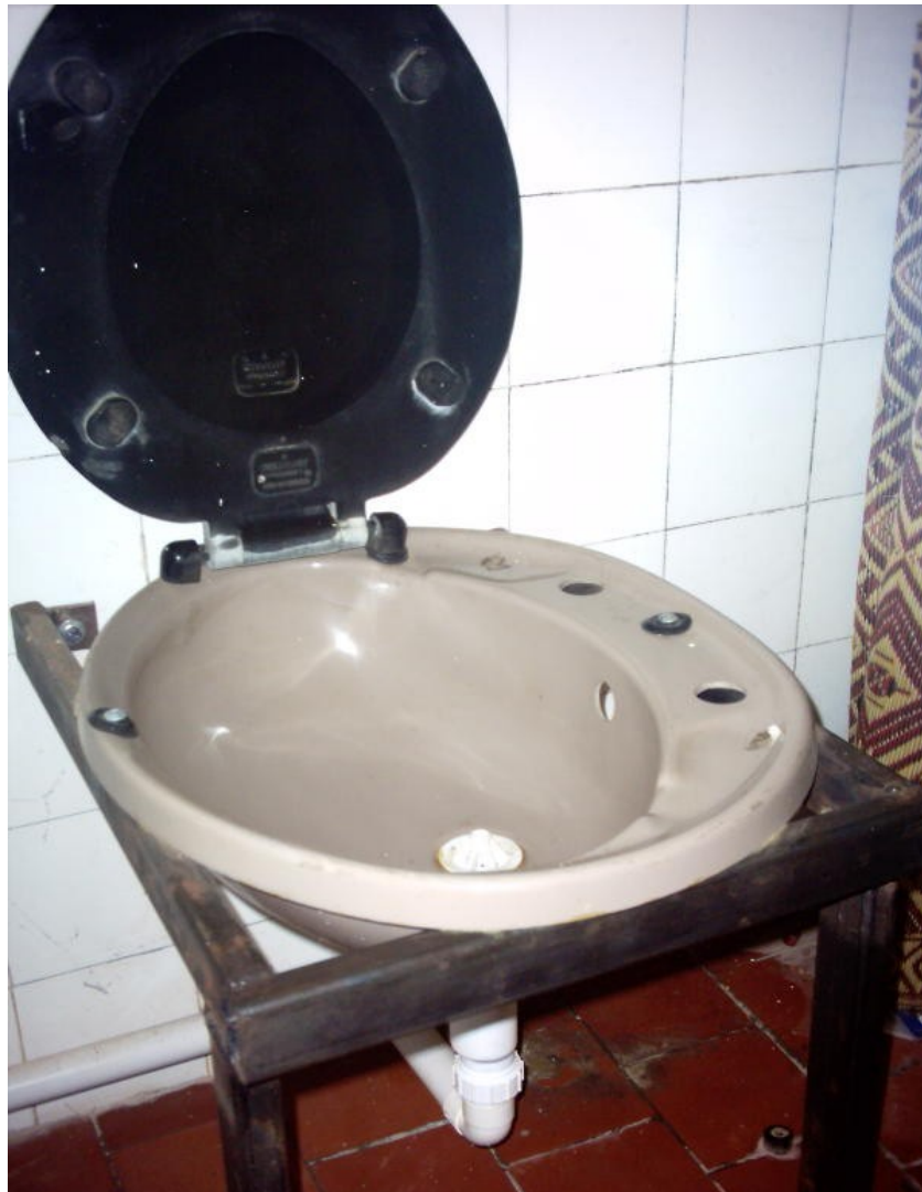
This unisex urinal consists of a seat and lid attached to a washbasin fixed to a home-made metal frame (although a bidet would be better). It has a normal waste kit with a Hepworth valve attached underneath.
