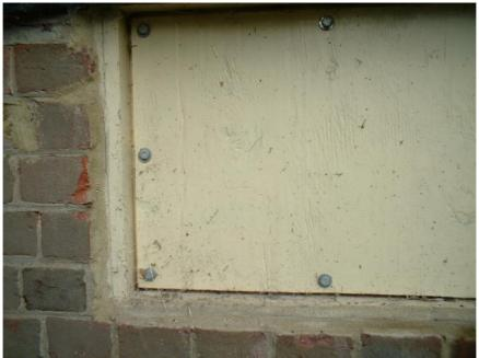
A hole has been knocked through the external wall for the hatch; coachscrews fix the hatch to the frame. The hatch can be removed, and the chamber emptied into a wheelbarrow with a long-handled shovel. The inside of the hatch is painted with bituminous paint to stop it rotting.
