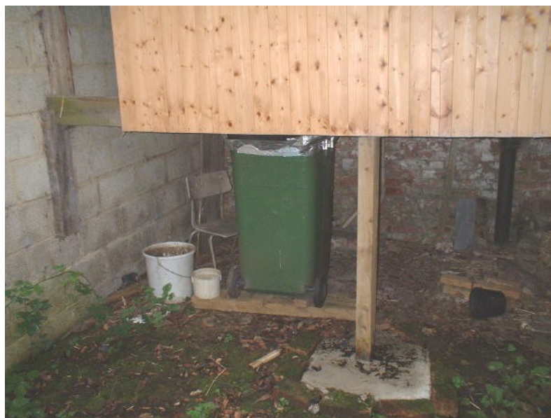
Wheelie-bin compost loo underneath a straw-bale extension (clad with tongue-and-groove).
