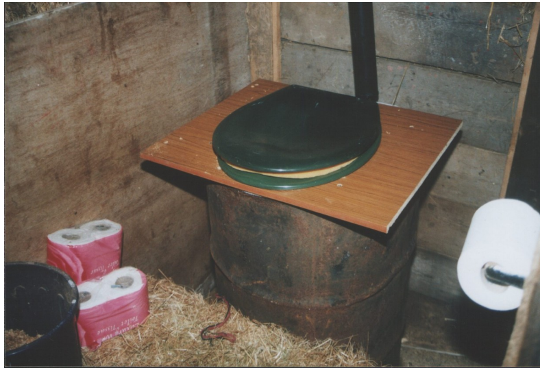
Temporary 'oil-drum' compost toilet, with vent pipe, and straw-bale steps.
