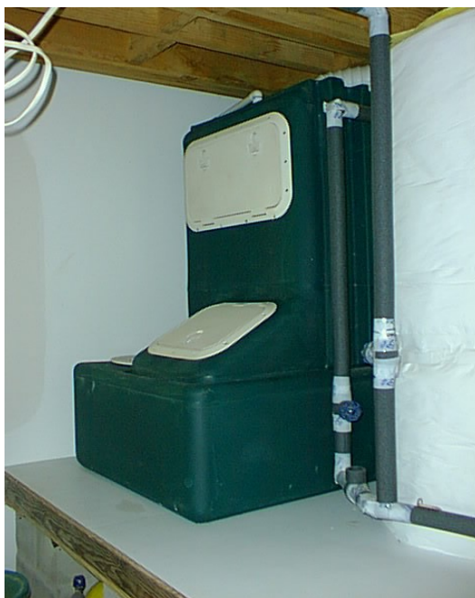
Composting chamber of a Clivus Multrum
