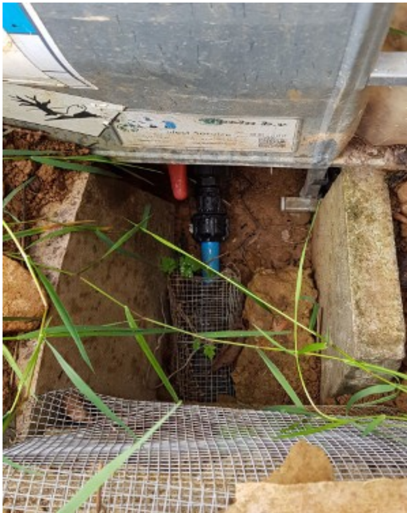
Urine leaves the IBC through 25mm MDPE pipe.
